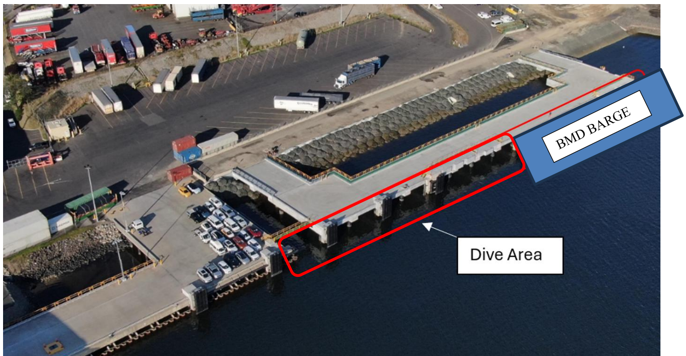
Berth 3 East Work Area
