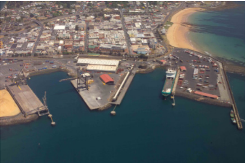
Aerial view of the Port of Burnie.
