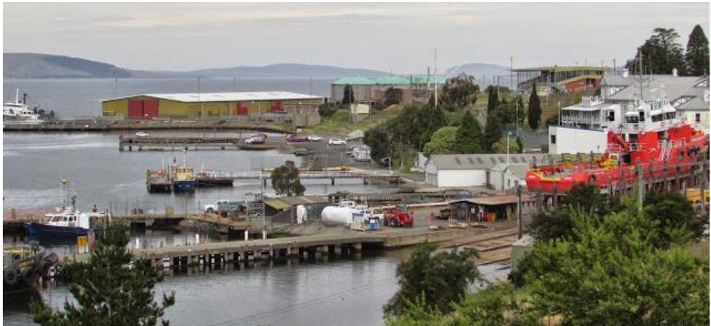
Figure 5 – Selfs Point bulk hydrocarbon unloading berth .
