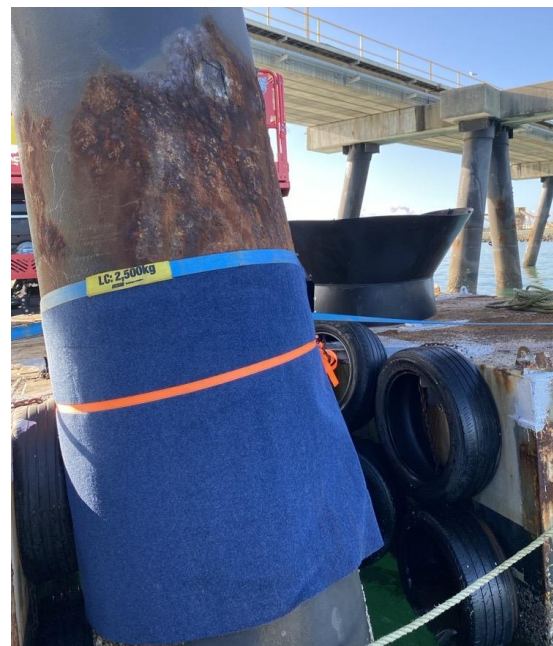
Figure 1b: Padding to help hold funnel from slipping down the pile
