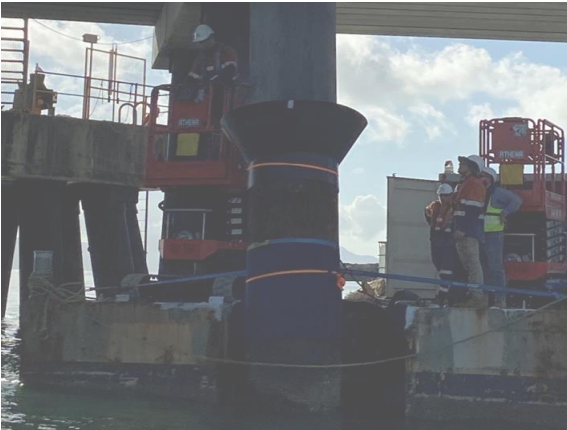
Figure 1c: Funnel on pile capturing waste from blasting activities
