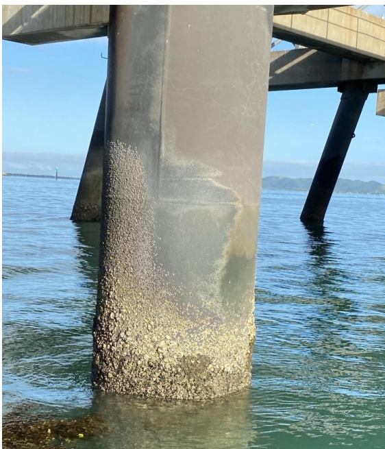
Figure 1a: Pile to be scraped
