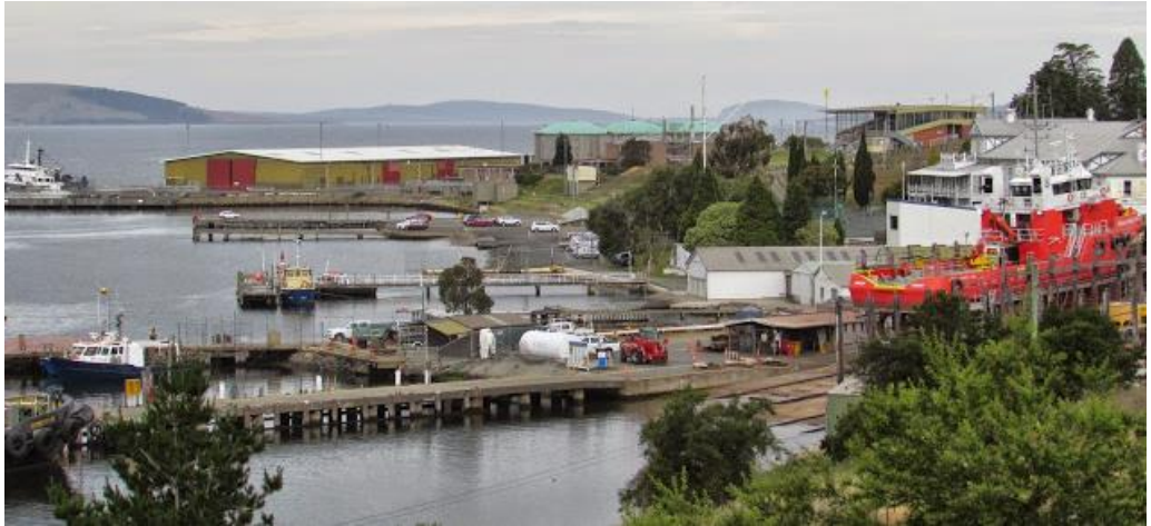
Figure 5 – Selfs Point bulk hydrocarbon unloading berth .
