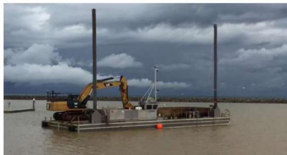
Self-propelled barge Constructor 3
