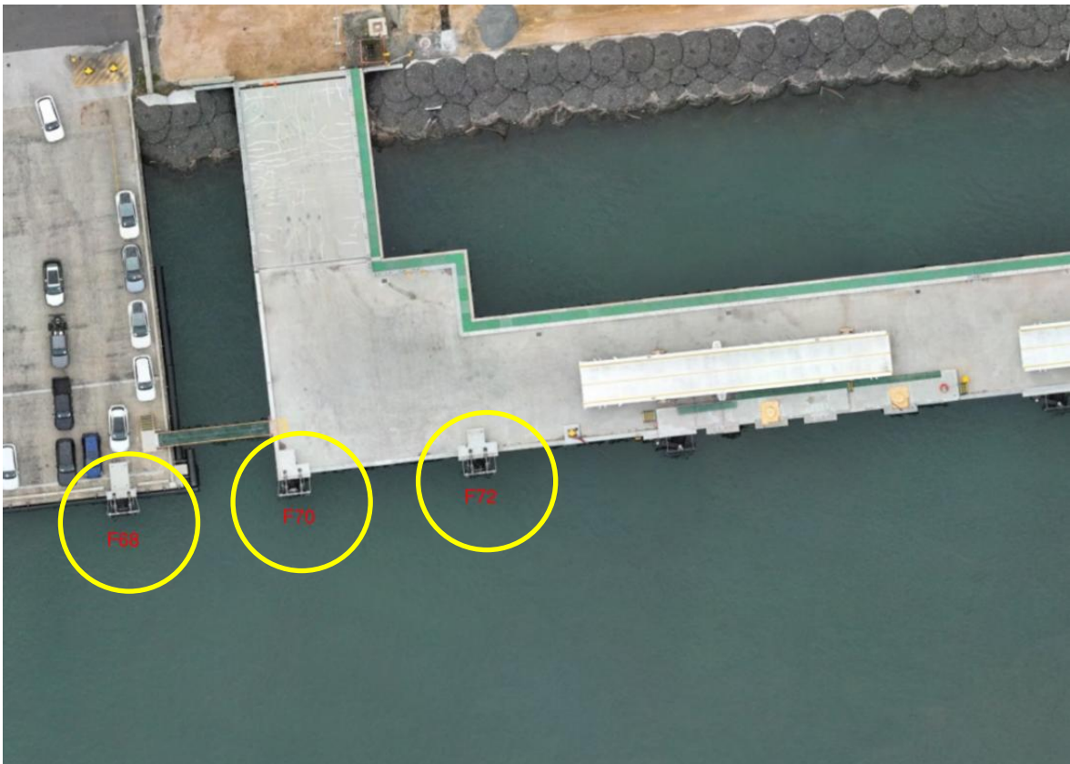
Berth 3 East Work Area
