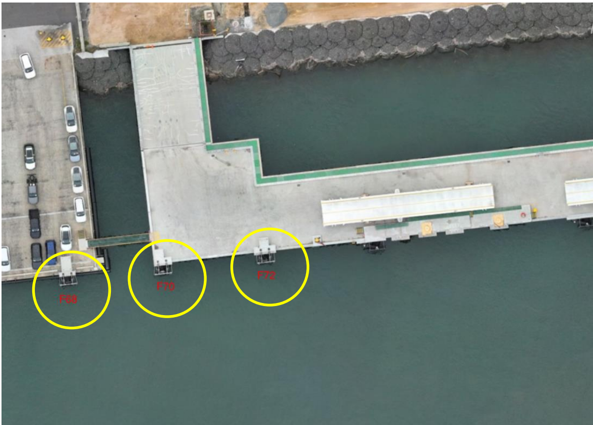
Berth 3 East Work Area
